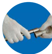
3. Marking pipe insertion length
